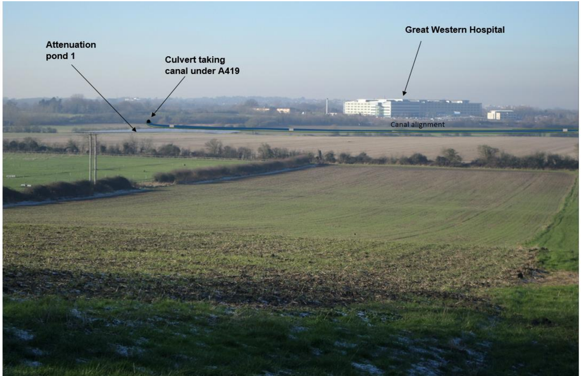
Figure 4 – View of canal through Liden Brook floodplain
