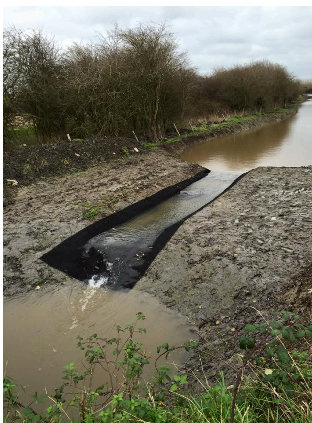
Western Section of canal completed - Studley Grange
