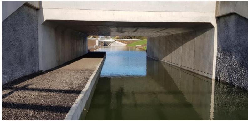
Completed A38 crossing
