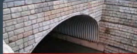
Attractive culverts can be achieved
