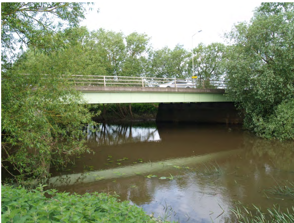
13 Challeymead (A350) bridge looking west
