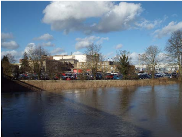
The CooperTires site (seen here with the river in flood) provides 25,000m 2 of land for regeneration, while retaining the tyre operation and existing employment
