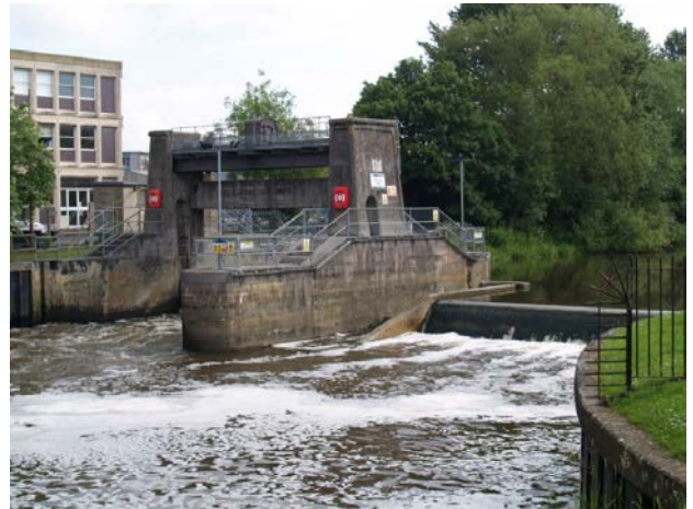
The existing weir and flood gate on the River Avon would be bypassed by a new lock (to the right of the photo), as well as a hydropower turbine and a fish pass
