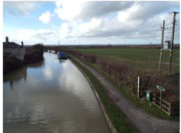
Site of proposed new junction with Kennet & Avon Canal at Semington - the Melksham Link would leave to the right
