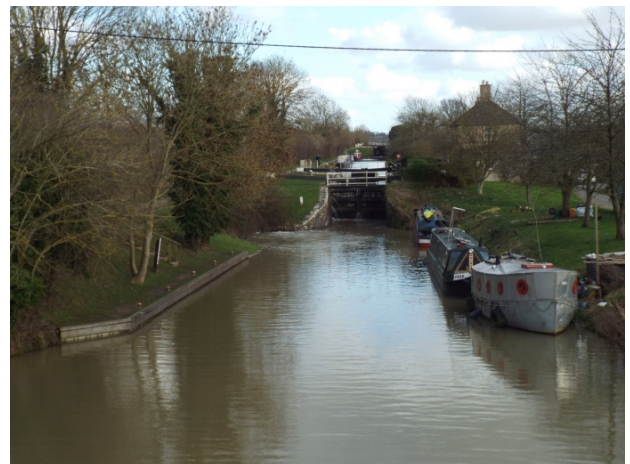
Typical canal locks on the Kennet & Avon at Semington show the type of environment that could be created by the new link
