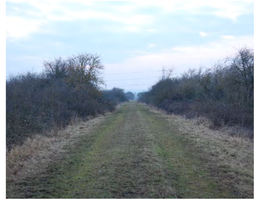
2. View along embankment
